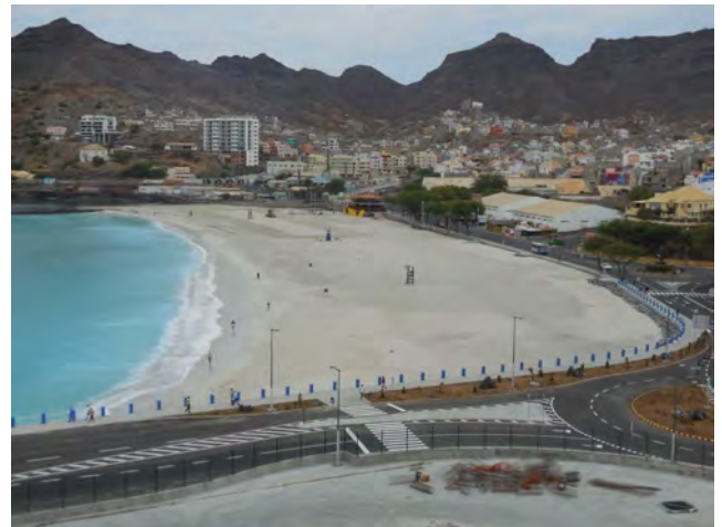
Laginha Beach after completion of sand filling
