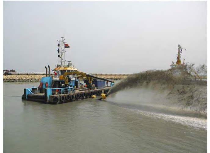
Dredging with DOP pump
